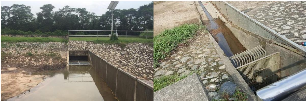
Figs. 8. A filtration system at the start of drain channels into the mangrove area.
