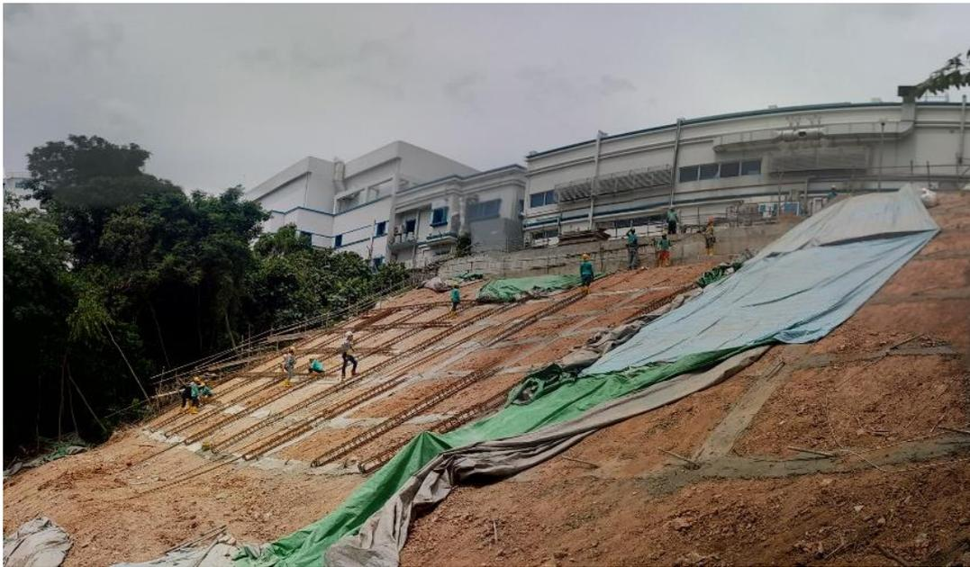
Fig. 5. Construction of grid beams in October 2016.
