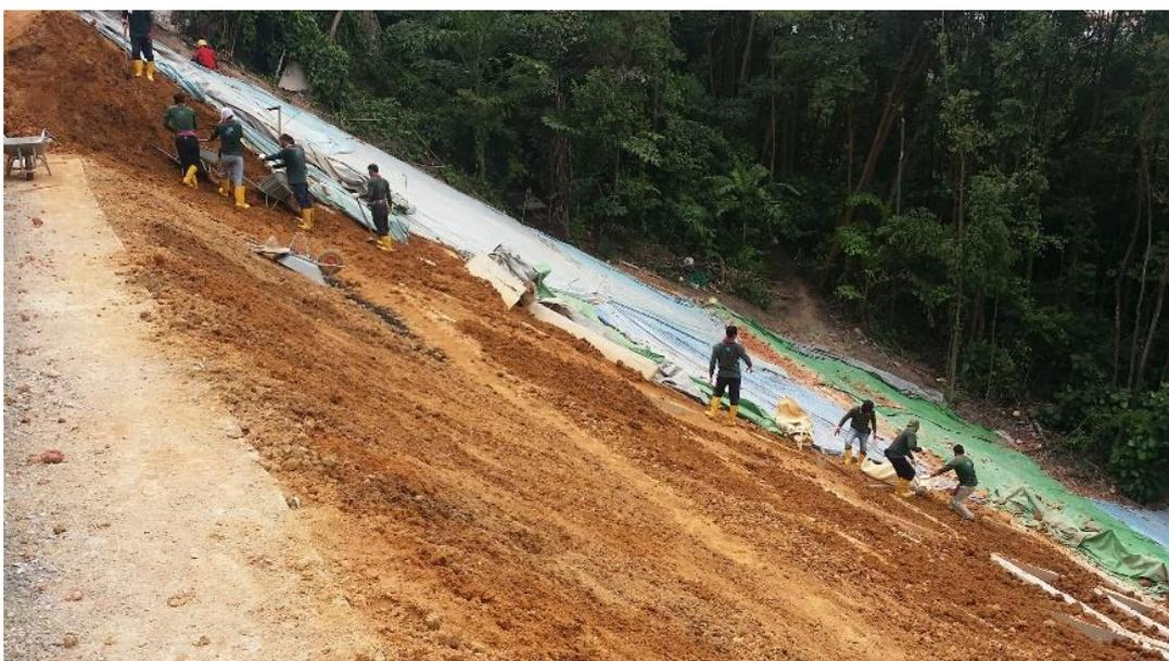
Fig. 6. Backfilling of soil in January 2017.
