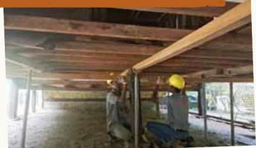
Replacement of flooring support
