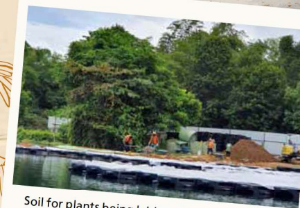
Soil for plants being laid on the bare floating platform that will be used for a new floating wetland
