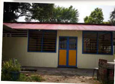
After completion in November 2019
