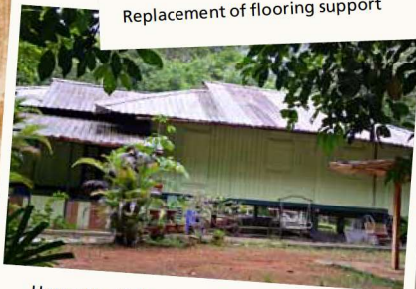
House No. 760D after replacement works
