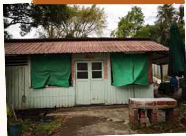
House No. 239 before repairs
