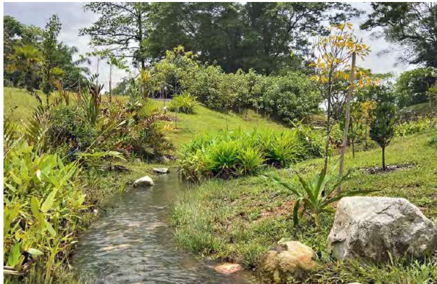
A concrete drain leading from Yuan Ching Road to Jurong Lake has been naturalised into a series of streams known as Neram Streams that channel stormwater runoff from the surrounding area.
