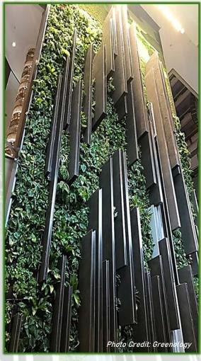
We developed and devised innovative ways to ensure the sustainability of an interesting mix of plants, through the use of our customised Greenology Vertical Greenery system, integrated irrigation and fertigation system.
