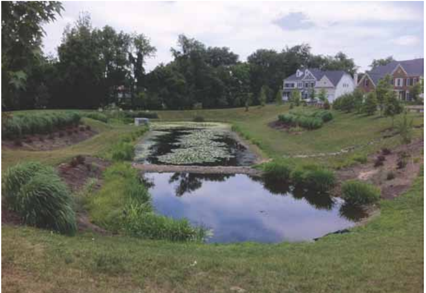
FIG. 5. A stormwater detention pond in a residential suburb of Baltimore (Photo: Chris Swan).
