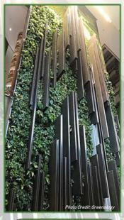
We developed and devised innovative ways to ensure the sustainability of an interesting mix of plants, through the use of our customised Greenology Vertical Greenery system, integrated irrigation and fertigation system.
