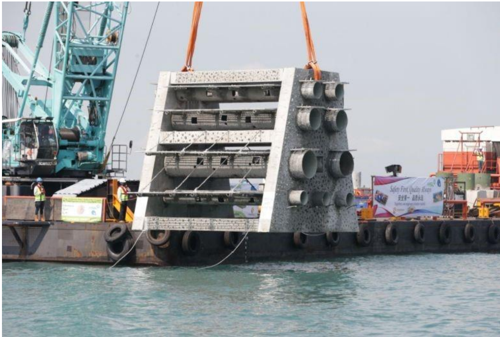
Figure 4 Reef enhancement structures that were placed in SIMP in 2018 (Source: Low, 2018b)
