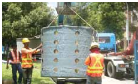
4. Installation of large container for street tree planting.
