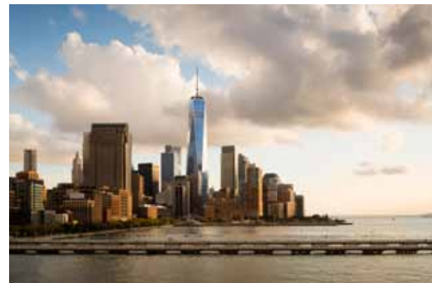
The Best Tall Building Americas went to One World Trade Center. The building's structure pays tribute to the first World Trade Center towers (Photo: James Ewing).
