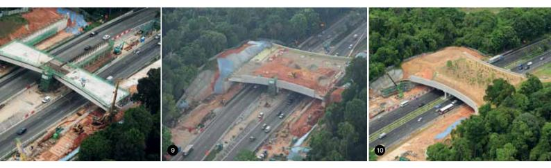
Shaped like an hourglass, the Eco-Link@ BKE is the first overhead ecological corridor in Southeast Asia. Extra effort was made to ensure undisrupted traffic flow along the expressway, while keeping the environmental footprint of the construction to a minimum.
