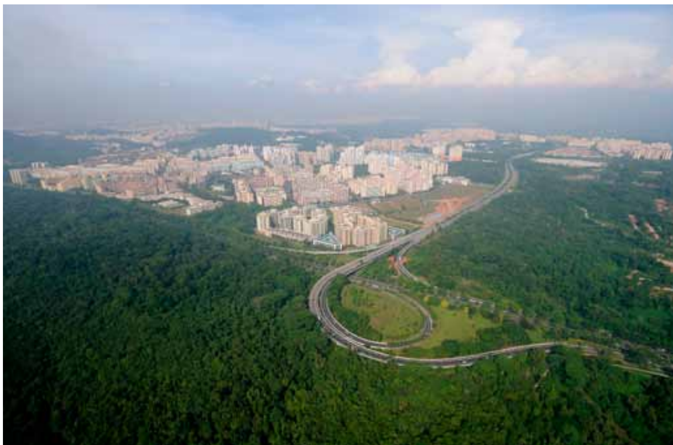
ABOVE Bukit Timah Expressway (BKE), where Central Catchment Nature Reserve lies on one side of the expressway, and Bukit Panjang Residential town sits on the other. The Singapore Index can be used as a planning tool for urban planners to designate protected areas and balance conservation and development (Photo: Wong Tuan Wah).
