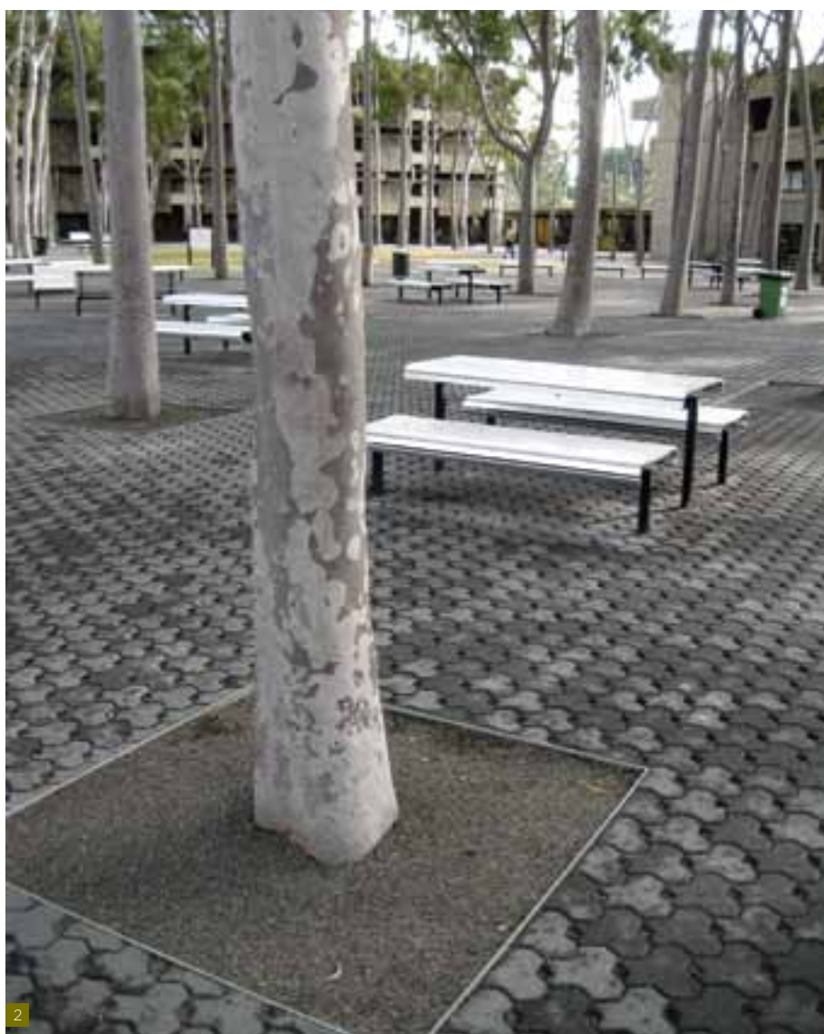
1. Permeable decking on a city sidewalk spans over uncompacted rooting soil, freeing trees to grow to full size.
