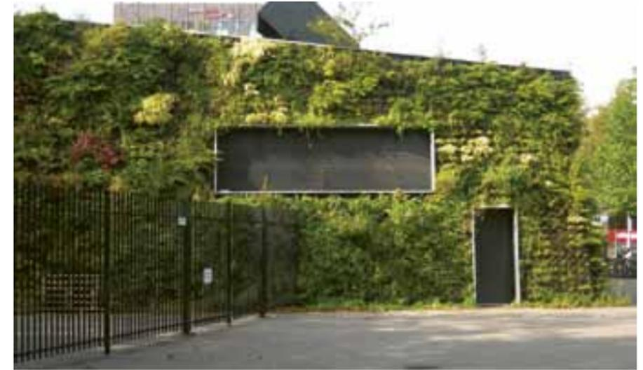
11. An example of a living wall system based on felt layers in Amsterdam, The Netherlands (see Fig. 2e for illustration).
