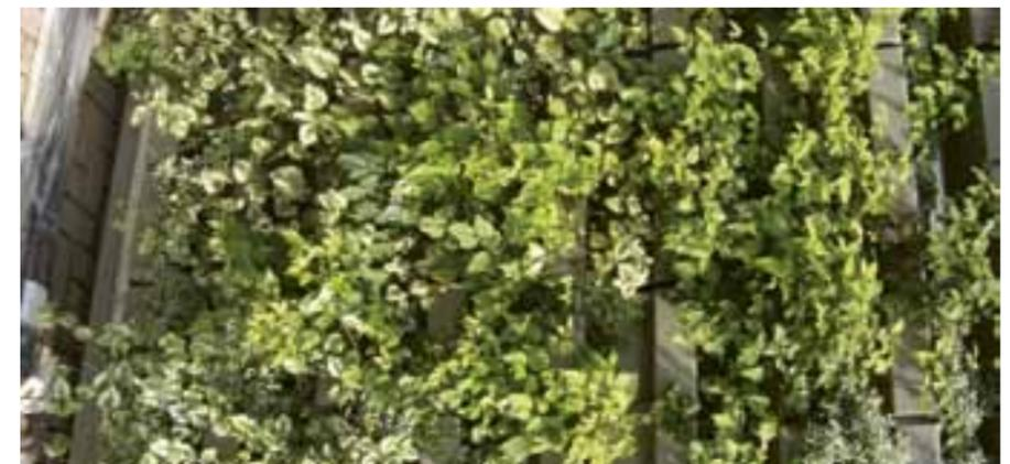
13. An example of a living wall system based on planter boxes in Delft, The Netherlands (see Fig. 2d for illustration).
