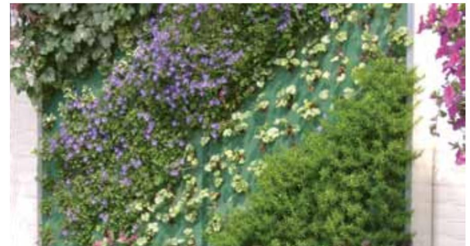
12. An example of a living wall system based on mineral wool in Utrecht, The Netherlands (see Fig. 2f for illustration).
