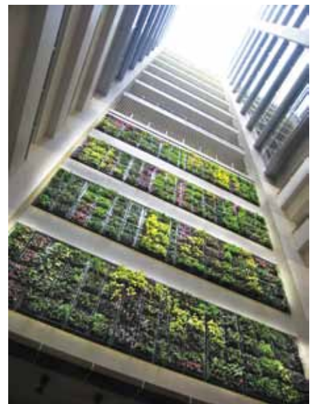
4. National University Hospital, an example of high-rise greenery with well-designed maintenance walkways (Photo: DP Architects Pte Ltd).
