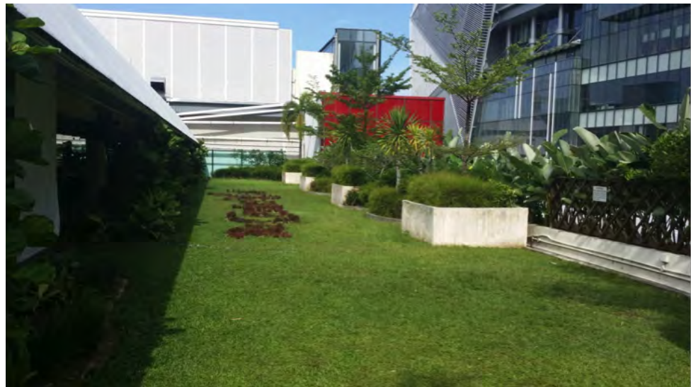
Intensive retrofitted roof garden
