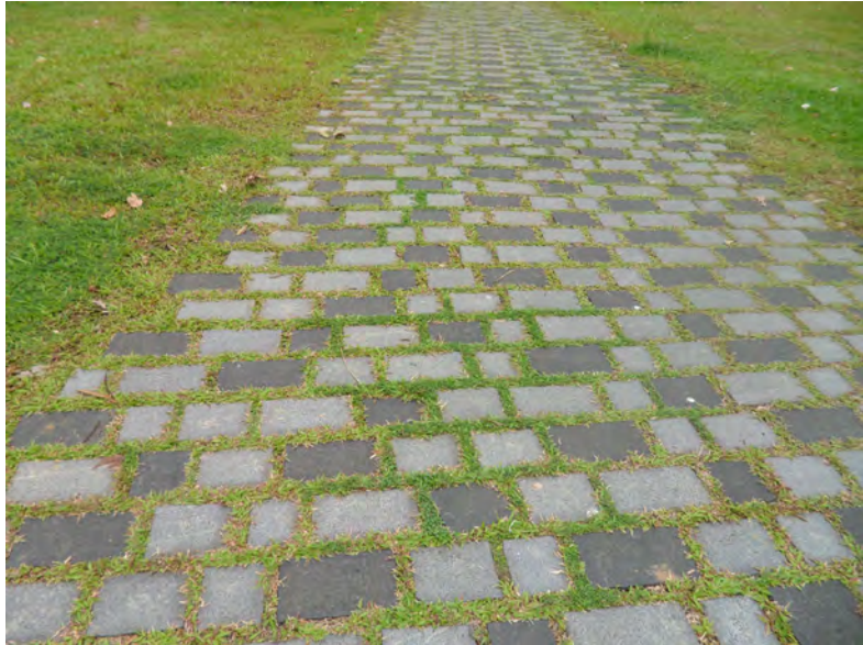
Avoid having grass in crevices to reduce maintenance
