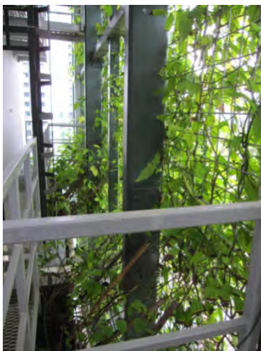
Tree House Condominium has a façade of vertical greenery, composed of climbing vines, with a back-accessed maintenance walkway. Maintenance from the front is kept to a minimum.
