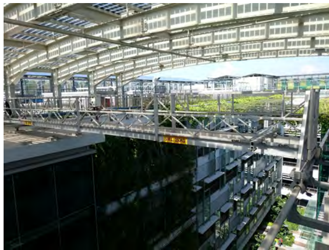
Sky trellis platform at JTC Cleantech Park One
