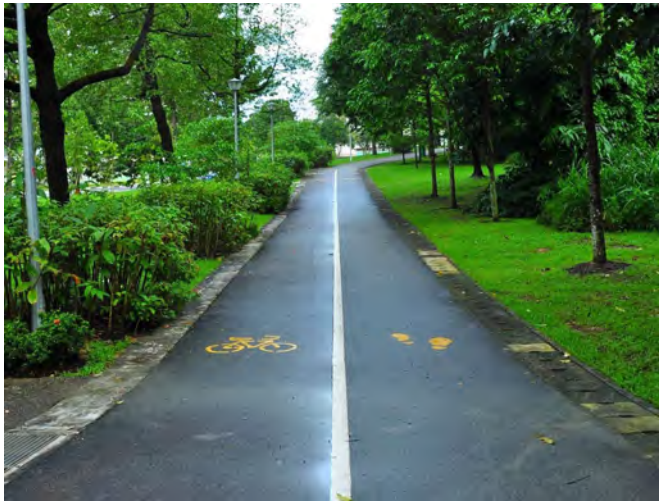
Asphalt is most suitable for cycling paths in parks and park connectors
