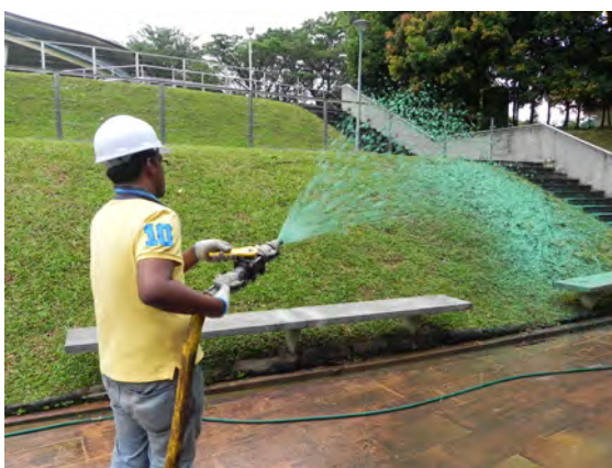
Hydrosprigging application using cocopeat mulch slurry
