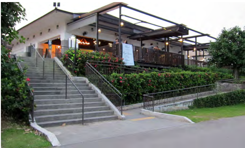
Handrails provided for staircase and ramp
