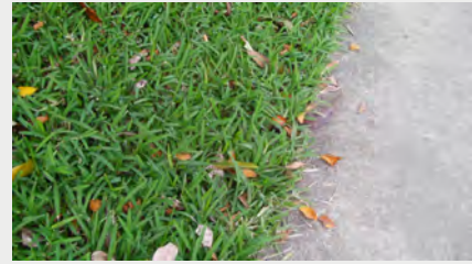
Properly reinstated grass should be lush, evenly graded and compacted and level with path or above it.
