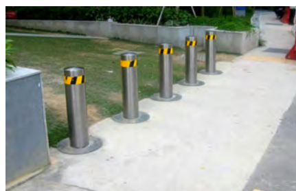
Reflective band on bollards helps improve visibility
