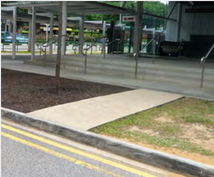
Mulch can deter people from trampling over the area and protect trees from soil compaction.
