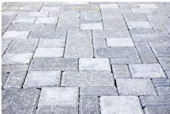
Pavers affected by tree roots are easily relaid
