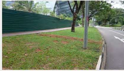
Poor reinstatement of grass after trenching creates uneven surfaces for the lawn.
