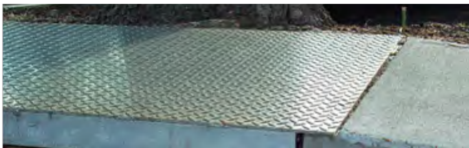
Bridges can be an alternative to root pruning — instead of removing roots, a pier-and-beam design can provide pedestrian access over the offending roots
