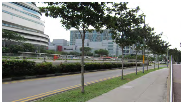
Roadside trees with minimal planting provision
