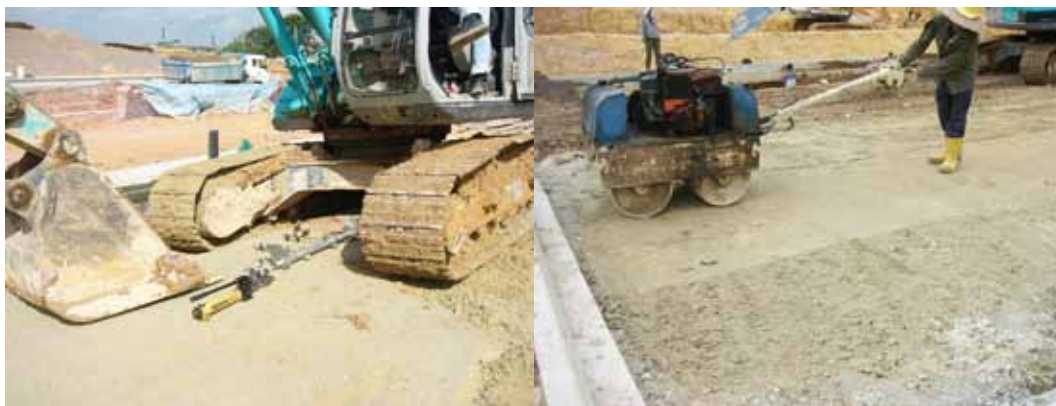
Fig 5. Load bearing tests conducted prior to the opening of the car park.
