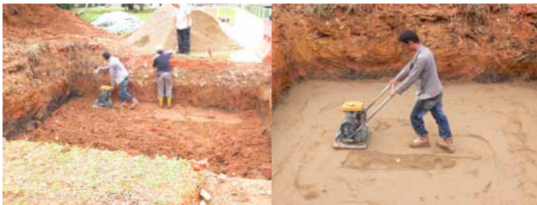
Fig 3. Setting up of tree pits at Springleaf Park to receive structural soil.
