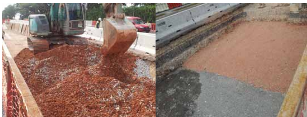
Fig 6. Installation of structural soil along Old Choa Chu Kang Road.
