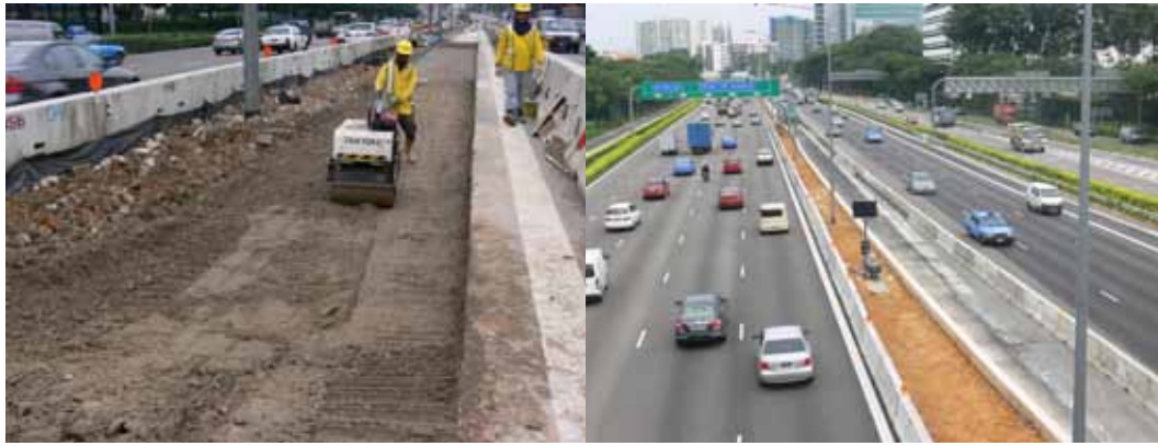
Fig 4. Installation of structural soil along PIE.
