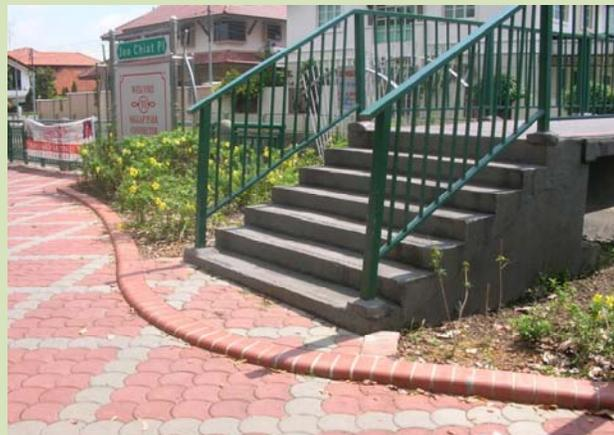
An irregular riser within a very long and consistent flight of steps can be especially disconcerting as it is totally unexpected.
