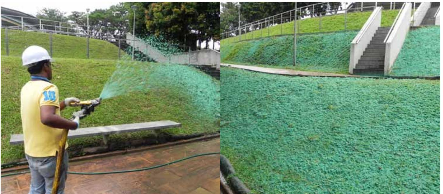
**Fig 1.** Hydroseeding to rehabilitate poor quality turf.
