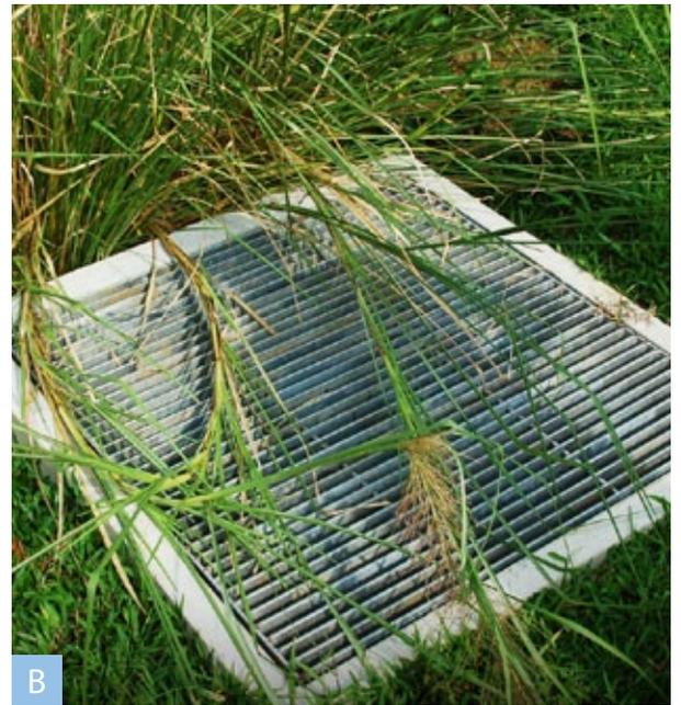
**Fig 3.** (A) The debris accumulated needs to be removed. (B) This outlet grate is not clogged, but vegetation and rubbish may continue to collect on the grate, causing water to spill into surroundings.
