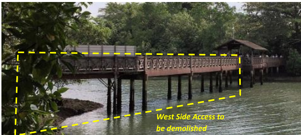
Figure 2-1: Existing Sungei Buloh main bridge
