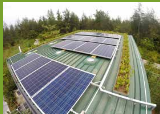
Solar panels and plantings on the roof of the zero-energy self-sufficient toilet
