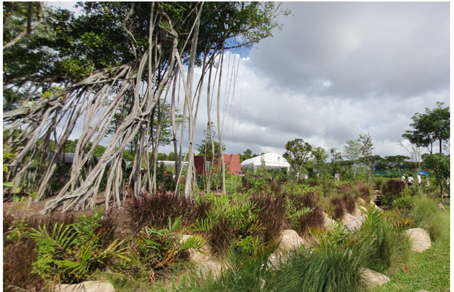
Naturalised drain at Sembawang Hot Spring Park
