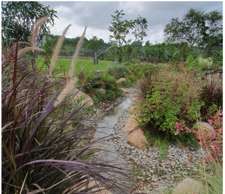
Naturalised drain with vegetation along the edges to help slow down run-off, and a gravel bed to allow water infiltration into the ground
