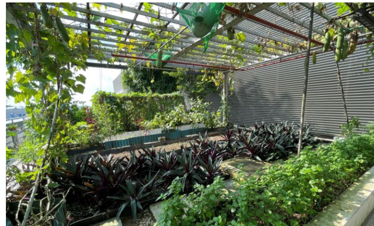
Yishun Community Hospital
