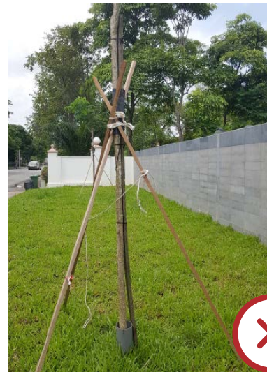
Untidy staking/ not firmly fastened to tree
