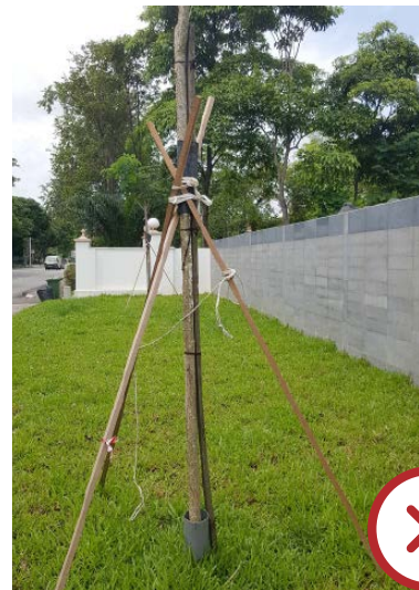
Untidy staking/ not firmly fastened to tree
