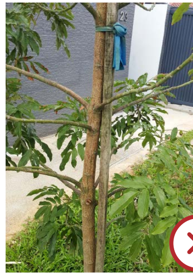
Improper staking (too close to tree)
