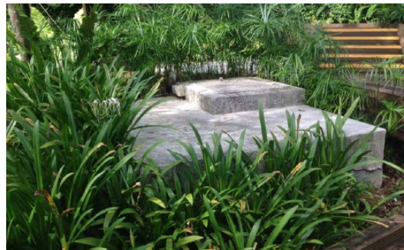
Water Bulk Meter
