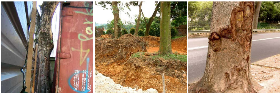
Lack of Tree Protection Zone
