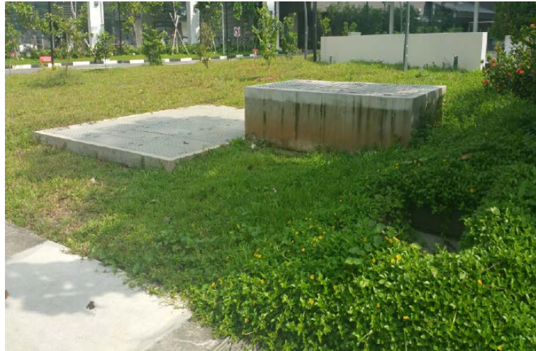
Bulk Water Meter
