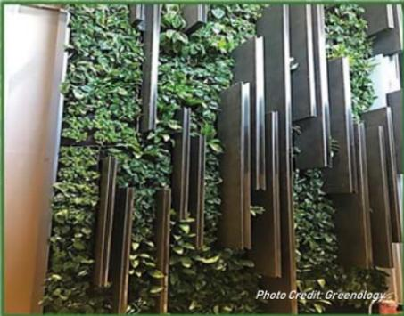
We developed and devised innovative ways to ensure the sustainability of an interesting mix of plants, through the use of our customised Greenology Vertical Greenery system, integrated irrigation and fertigation system.
