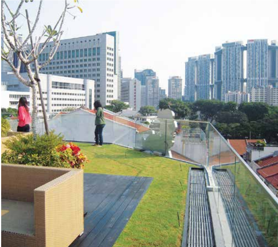
Safety barrier along the perimeter of a rooftop garden.
