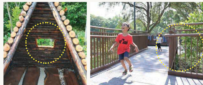
Figure 53. Examples of areas to check for entrapment hazards in a playground.
