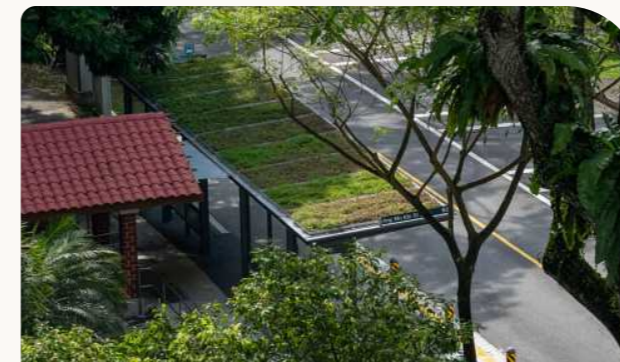
Studies have shown that green roofs, such as those found at select bus stops in Singapore, can reduce ambient temperatures.
