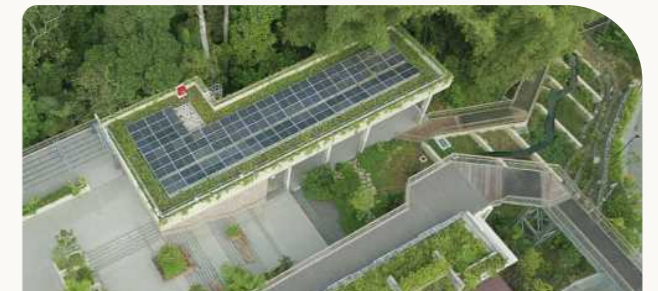
Energy harvested from the photovoltaic solar panels installed around Rifle Range Nature Park exceeds the expected annual operational energy consumption of the site, making it a net positive energy Nature Park.
