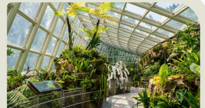
The spectrally selective glass in the Sembcorp Cool House maximises light penetration to promote plant growth.
