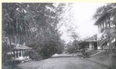
On the left, the original 1882 office-cum-Herbarium, now called Ridley Hall. Distant right, the first single-storey Herbarium built in 1905. This photo, dated 1922, shows the simple tiled roof that replaced the original ornate one.
