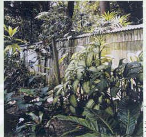
The wall near the Aroid Garden. Some marks are caused by snail grazing, others by circular growth patterns of algae.
