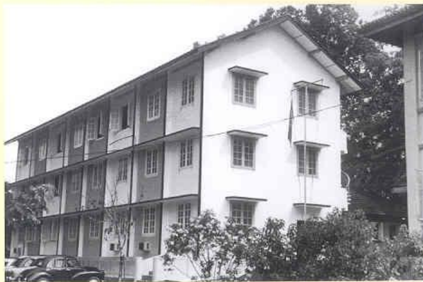
The third three-storey Herbarium completed in 1964.
