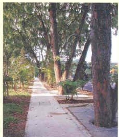
Roadside planting at the newly diverted Cluny Road. The large angsa trees ( Pterocarpus indicus ) have been preserved by constructing air wells around their bases.
