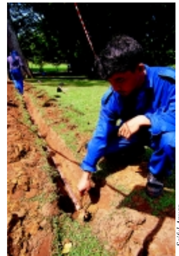
Installing the grounding system to complete the Lightning Protection System.
