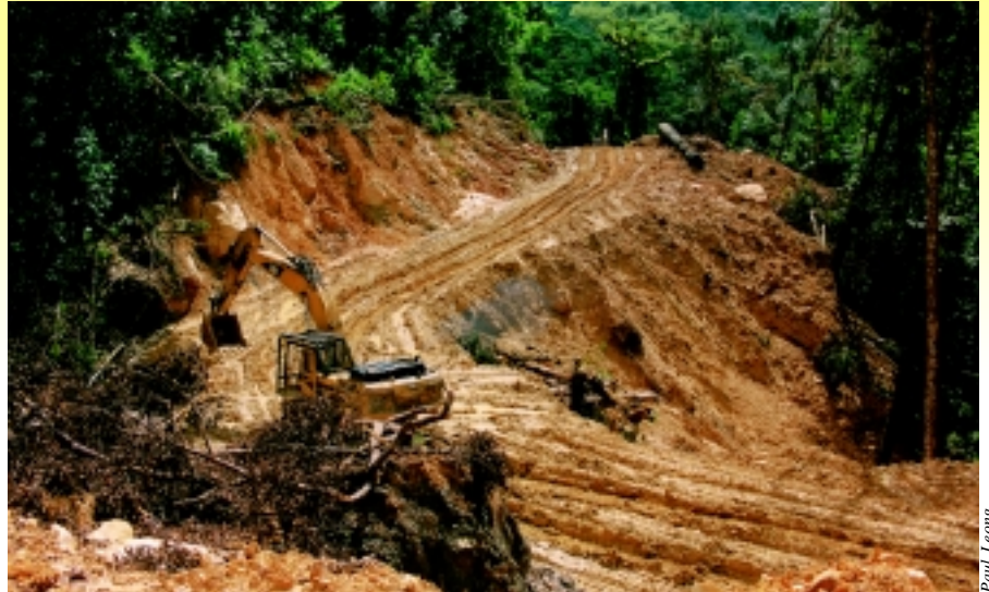
Logging roads caused landslips, severe erosion and siltation.
