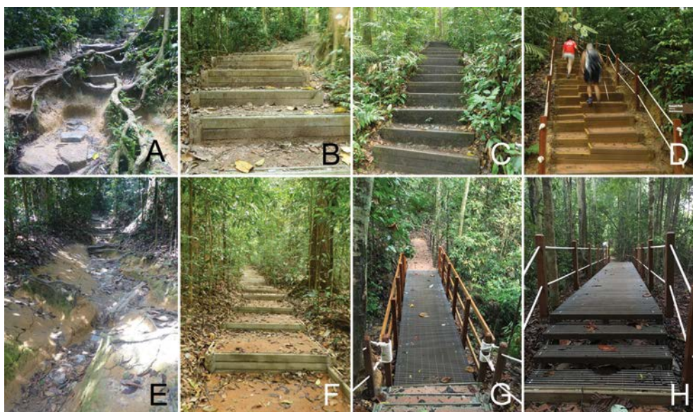
Fig. 10. Some of the trail repairs done by BTNR forest management during the forest closure. A. Dairy Farm Loop in January 2014. B. The same trail in July 2016 after repairs were made to control erosion. C. Summit Trail in Aug 2014. D. The same trail in Aug 2015, after enhancements were made to the steps. E. Catchment Path before repair in February 2014. F. The same path in July 2016. G. Broadwalk were constructed at various areas to minimise visitor impact to muddy stretches. H. Another broadwalk at the Dairy Farm loop area. (Photos: C. Chia).
