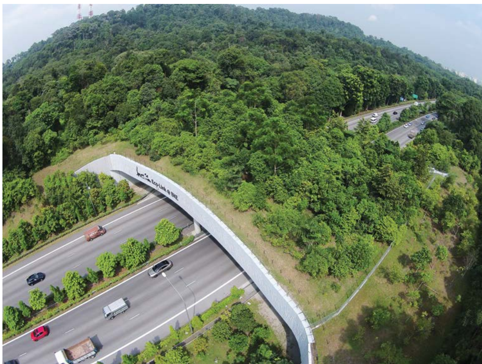
Fig. 2. An aerial photograph of the Eco-Link @ BKE (Bukit Timah Expressway). (Photo: T.W. Wong)
